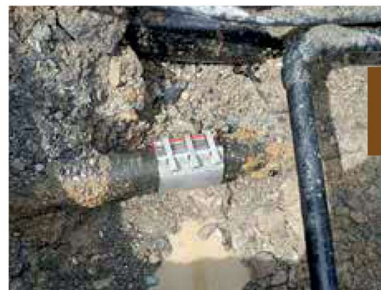
Damaged area on a pipe; quickly and reliably sealed with a STRAUB-REP-FLEX coupling.
